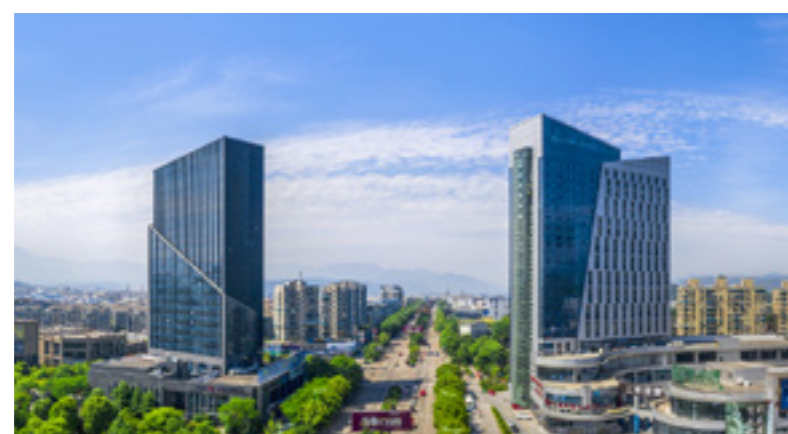
Lishui Economic and Technological Development Zone Management Committee Building--Immune architecture innovation demonstration project
