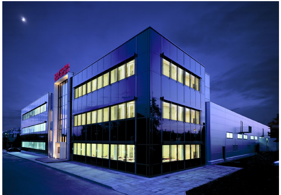
AIXTRON Production and Headquarters in Herzogenrath/Aachen, Germany
